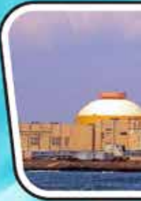
Kudankulam Nuclear Power Plant
