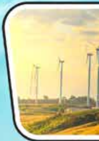
Muppandal Wind Farm
